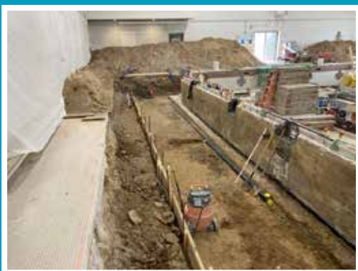
TRENT UNIVERSITY RENOVATION
