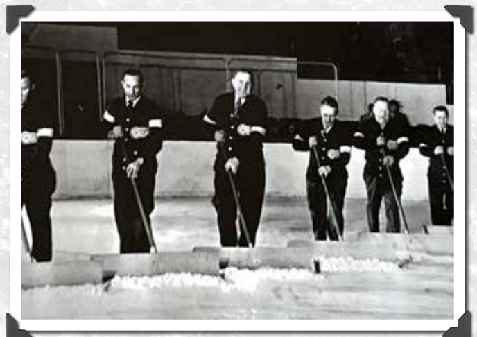
Lounging on the Shovel. In the pre-Zamboni ice resurfacer days, a tractor first swooped by with a giant blade to scrape the top of the ice before a gang of shovelers scooped up the shavings.
