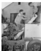
This was an early attempt to build a self-propelled resurfacer and in a 1964 patent lawsuit, Frank designated this unit as his experimental Model No. 3.
