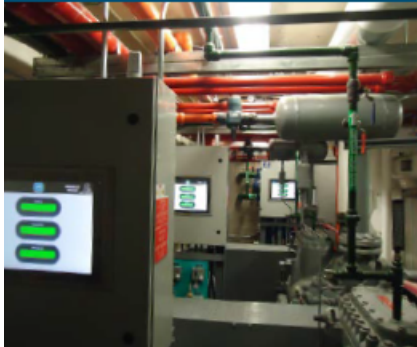
"Smart" low-charge ammonia/glycol system at Covent Garden Market Rotary Rink, London, Ontario
